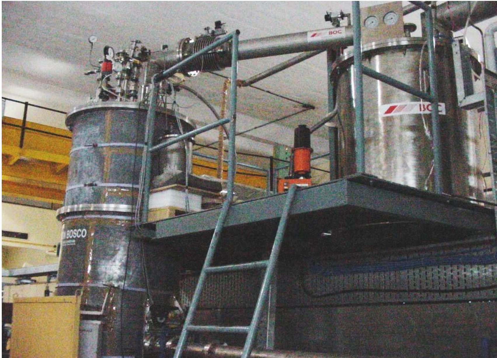
Superbuncher cryostat in beam line connected to the valve box
