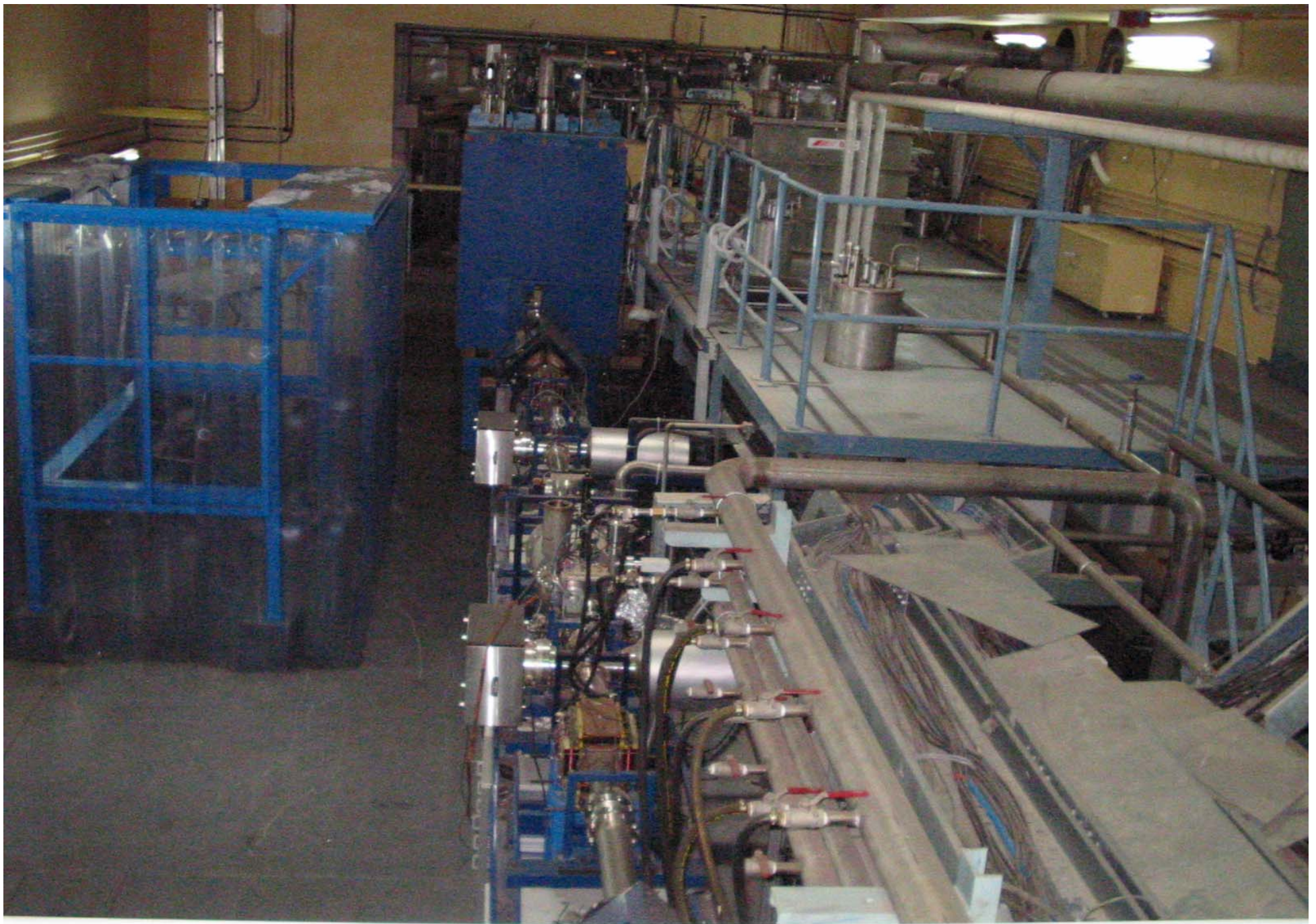
Linac Module with Beam Line and Cryogen distribution lines
