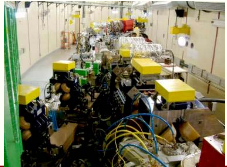
Transport Line-3 Joining on to Indus-2
