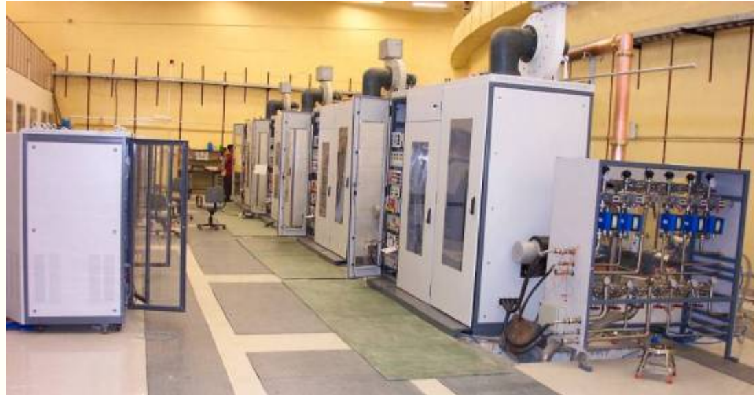
Indus -2 RF Power System
